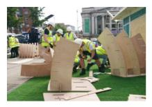
The Social Shell was completed in July 2019. From design to build, the pavilion took just over a year, with the help of a multitude of organisations and industry professionals. The project was cut from 61 sheets of Performance Plywood using CNC routers. The design minimised work on site, with only one site adjustment required, so that the pavilion could be constructed from a flat pack of parts in a single day and transported to different locations with minimum effort.
