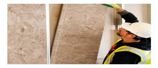
Pattress Plus is designed to provide support for fixtures and fittings in non-structural dry wall partitions. The product is an engineered OSB/3 panel incorporating a continuous recess, designed to accommodate 'C' shaped metal studs used in the construction of plaster board partitions.
