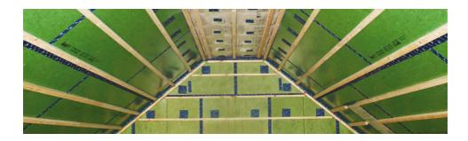
Propassiv is a structural OSB panel with intergrated vapour control and air barrier properties for use as structural sheathing in timber frame structures.
