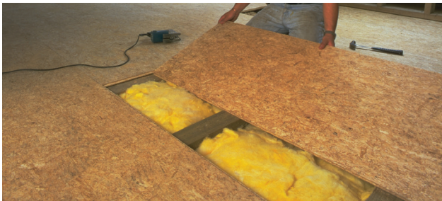
Figure 3: OSB panels used as flooring Photo: Wood for Good
