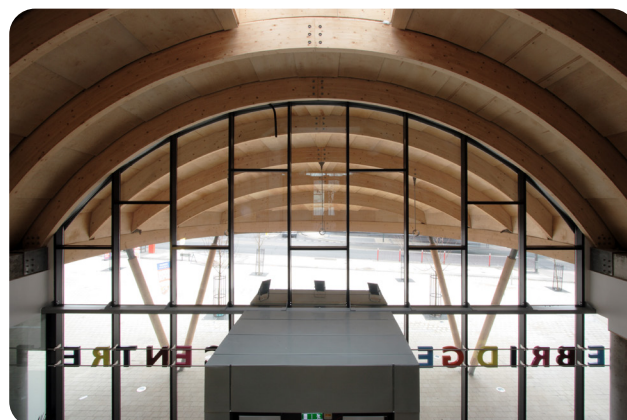
Figure 1: Woodstain finished plywood soffit lining at The Stonebridge Hillside Hub, West London
